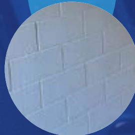
Block Works & Brick Walls
